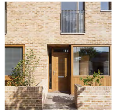
Front gardens provide defensible space
