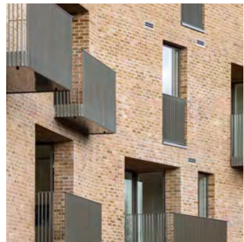
Balconies overlooking entrance route and park activities
